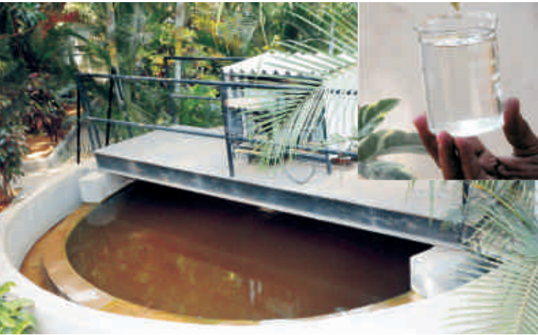
The clarifier at the canteen effluent treatment plant in Bangalore, which recycles and reuses domestic waste water.
