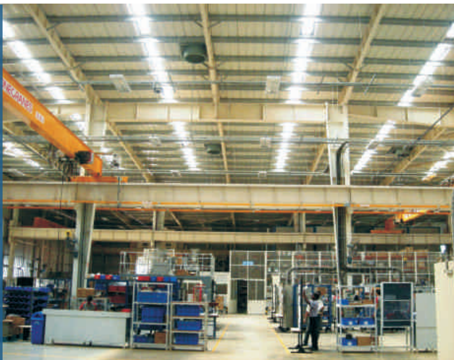
The skylights installed on the roof of the Verna Plant ensure optimum usage of sunlight.
