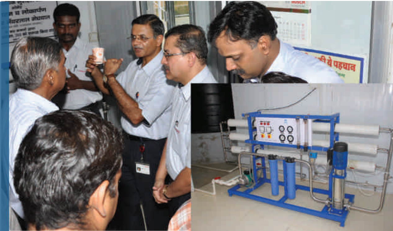
Bosch's Jaipur Plant has set up a Reverse Osmosis plant at the Government Industrial Training Institute and another one at Goner village.
