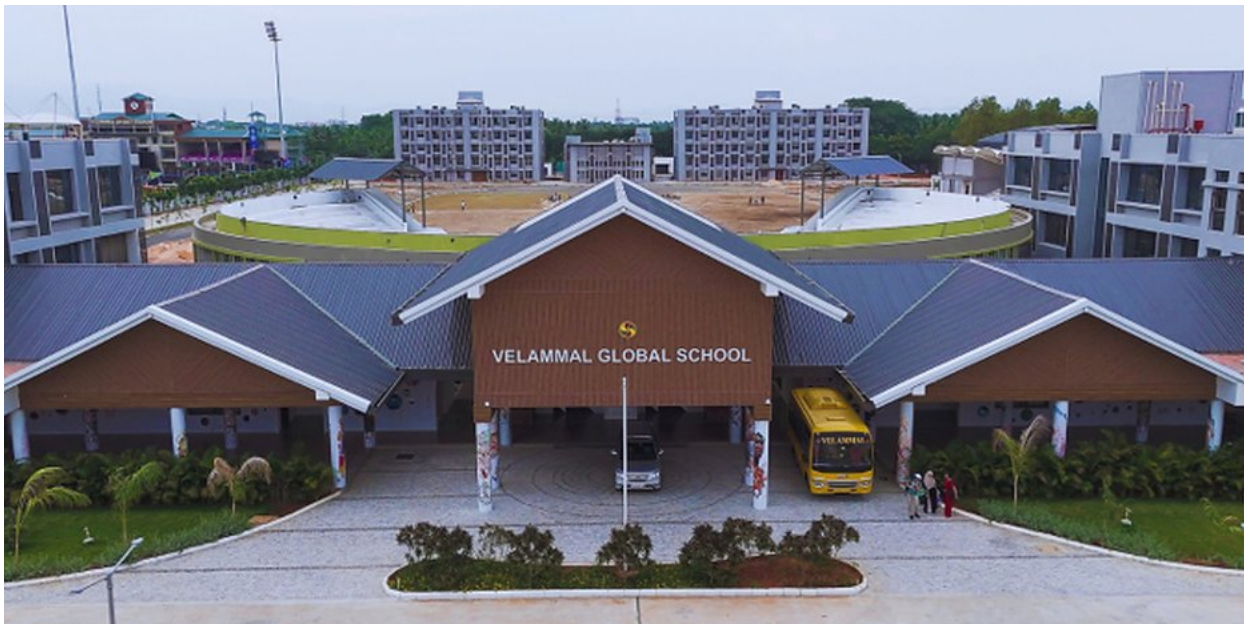
VRF and ducted systems at Velammal Global School, Madurai
