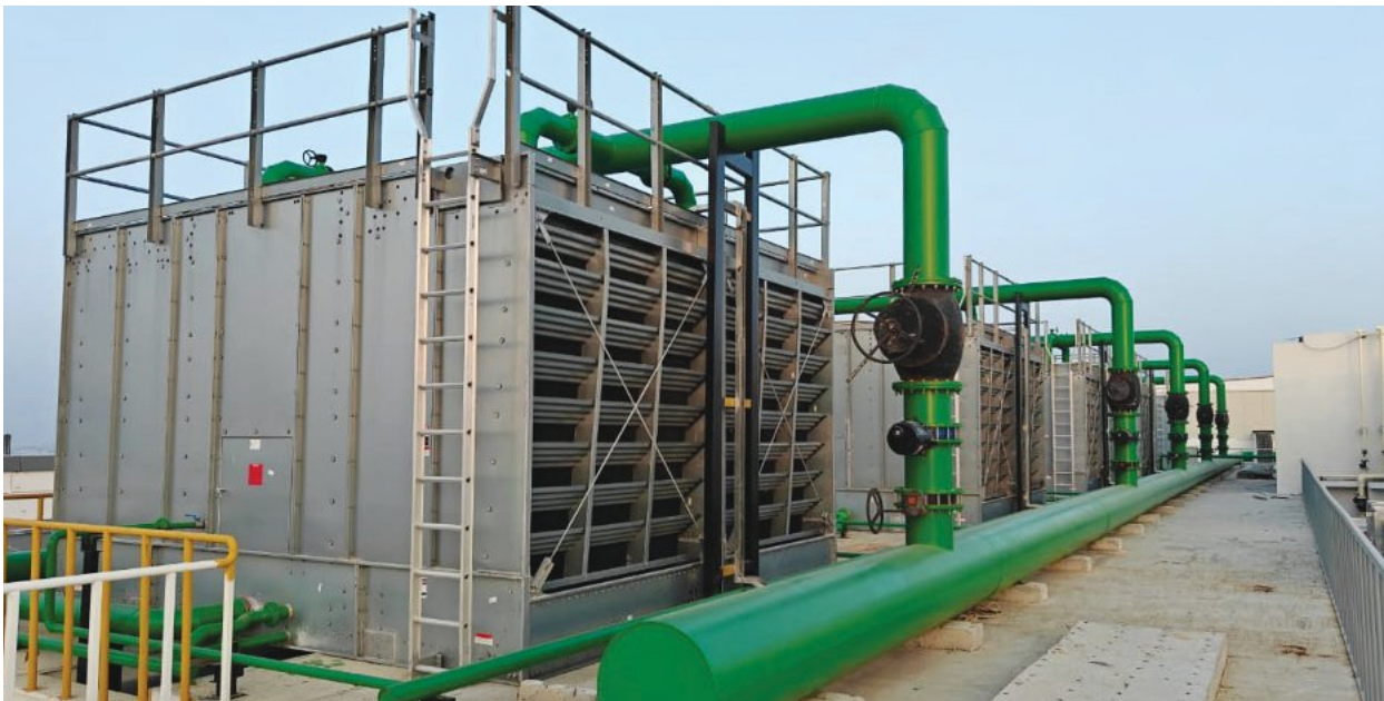
Enabling efficient living spaces with MEP works for Garden City Verde, Bengaluru
