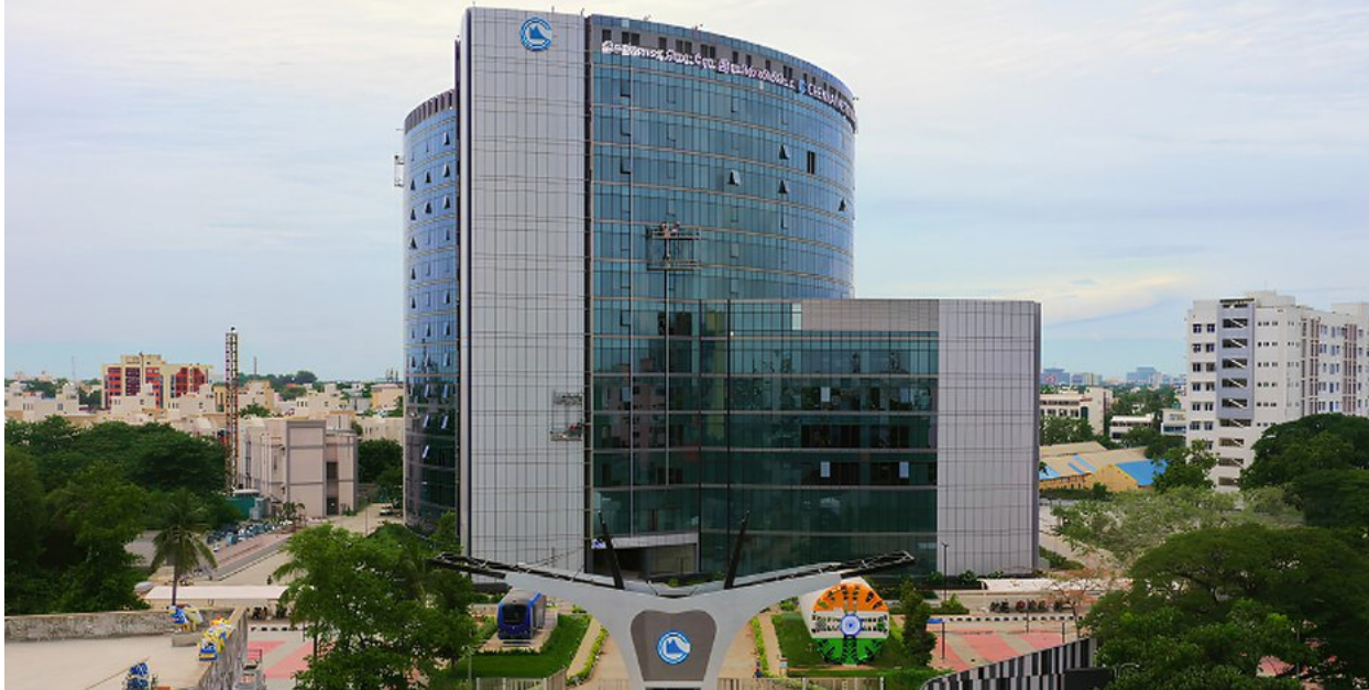
Screw chillers at Chennai Metro Rail Corporation
