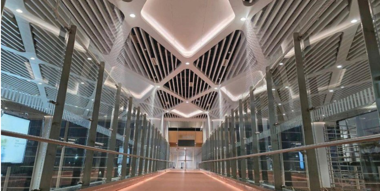
Enhancing passenger comfort through HVAC works at Noida International Airport
