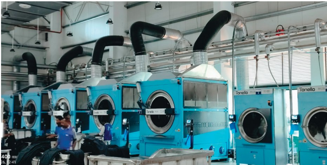
Facilitating efficient operations with MEP works for Trimetro Factory, Bhubaneswar, Odisha
