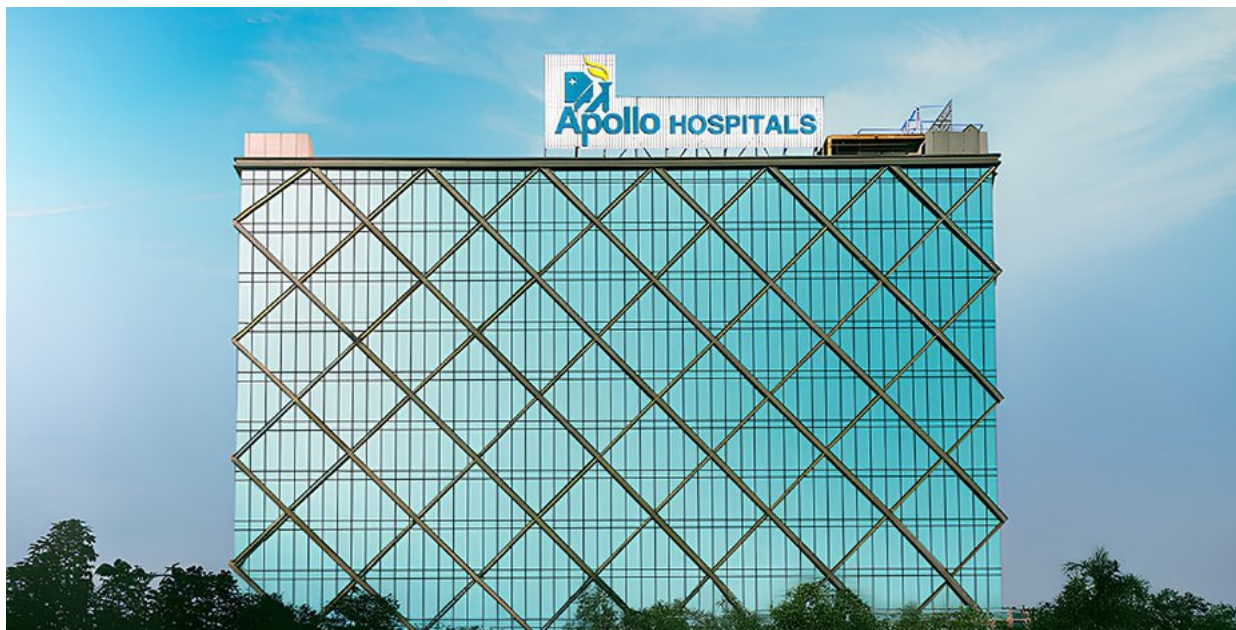
VRF and ducted systems at Apollo Hospital, Hyderabad
