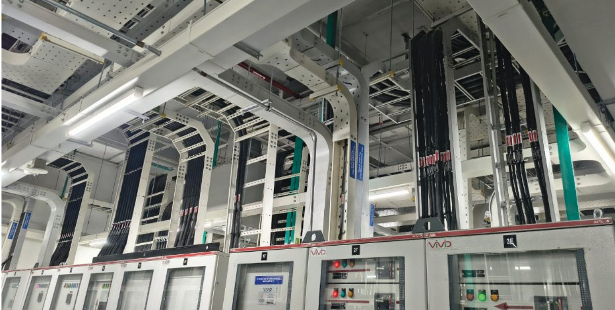
Advancing digital infrastructure through CSA & MEP works for the 24 MW STT Data Centre, Pune
