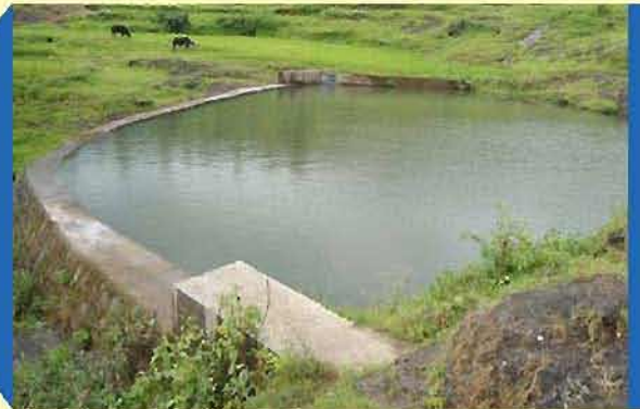
Rainwater Harvesting in Mokhada
