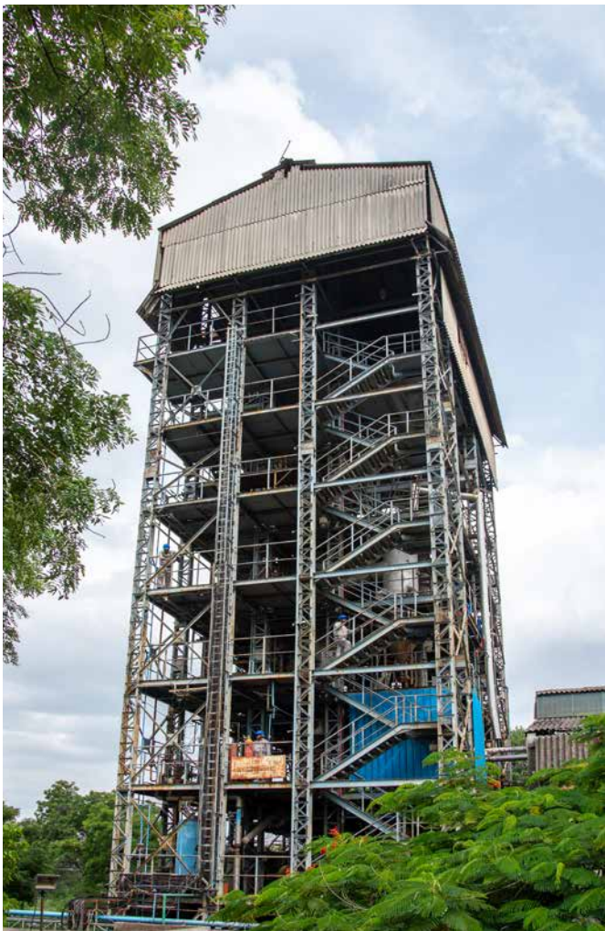
BHEL developed coal gasification facility in Hyderabad
