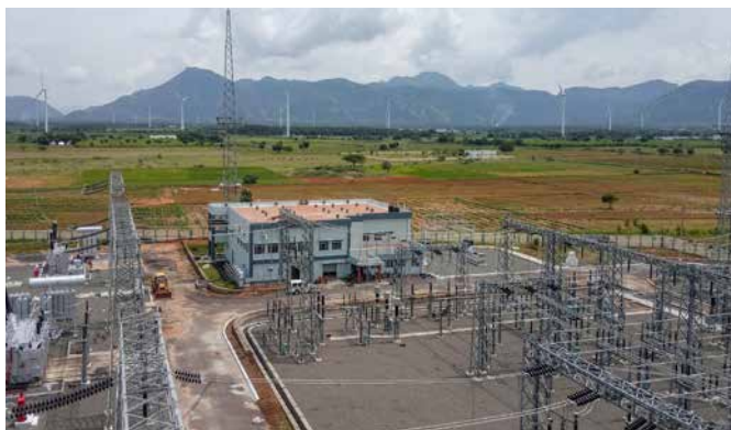
Thappkundu Substation (400kV - 9 bays, 110 kV - 12 bays) for TANTRANSCO commissioned by BHEL in October 2018
