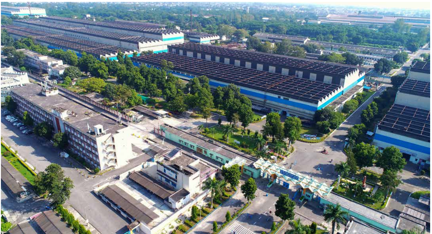
Heavy Electrical Equipment Plant (HEEP), BHEL - Haridwar
