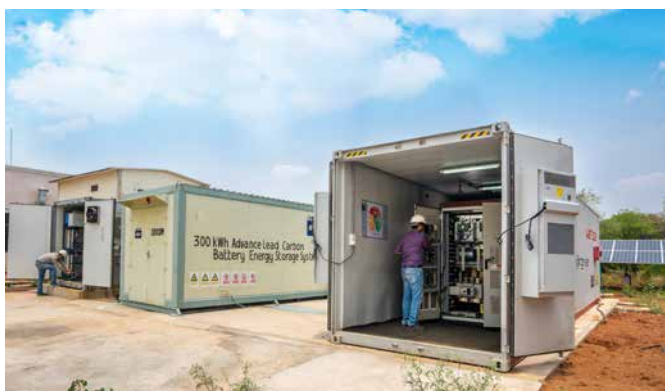
1 MWh grid-connected Battery based energy storage system (BESS) designed and developed by BHEL, installed at Corp R&D, Hyderabad
