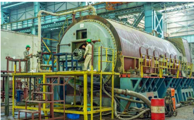
800 MW Generator testing at BHEL's Haridwar plant
