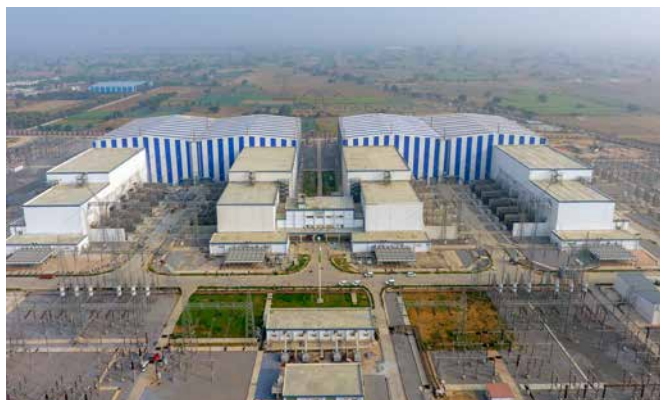
Aerial view of world's largest \pm 800 kV multi-terminal HVDC project (North-East to Agra), supplied and commissioned by BHEL
