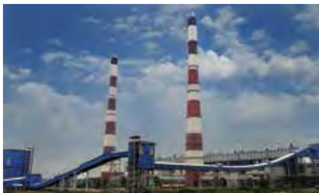
Unit-6 (150 MW) of Hindalco Industries Ltd.- Aditya Aluminium commissioned by BHEL
