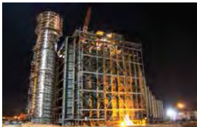
350 MW Yelahanka gas-based project for which BHEL won the 'Best Construction Project' award for safety from Karnataka Government
