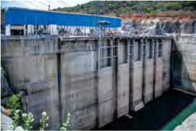
5x30 MW Mahatma Gandhi Kalwakurthy Lift Irrigation Project, Telangana, set up by BHEL
