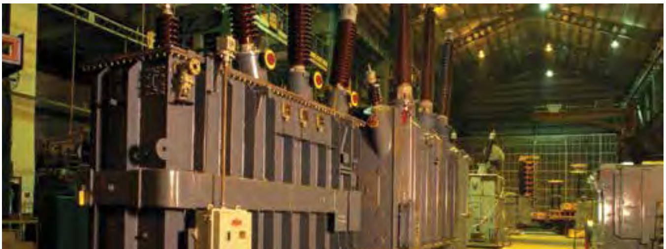
Transformer shop at BHEL, Jhansi
