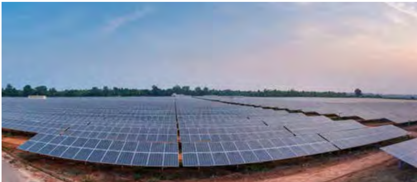
10 MW grid connected solar power plant at NLC township, Neyveli commissioned by BHEL
