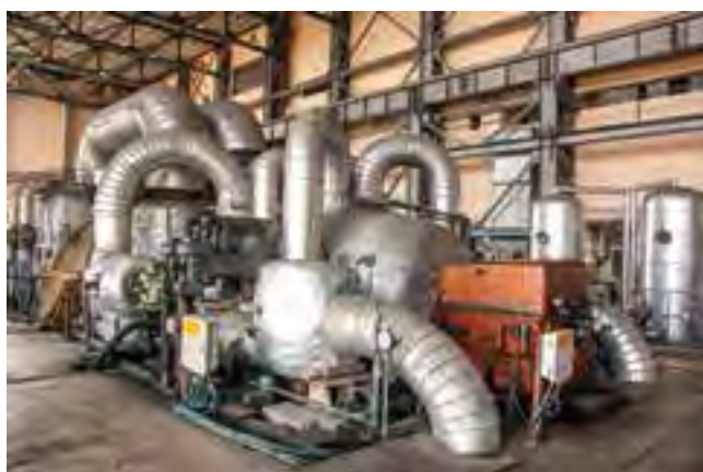
R&M of Barauni Unit 7 (110 MW) undertaken by BHEL
