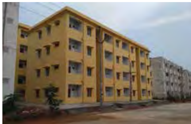
Model flats constructed by BHEL in Vizag, Andhra Pradesh for families affected by Hudhud cyclone
