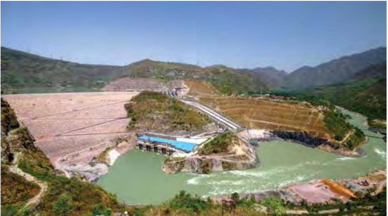
4x200 MW Koldam HEP commissioned by BHEL
