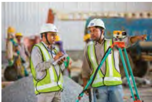
BHEL engineers at work on site
