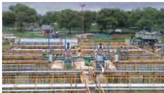
Membrane Bio-Reactor (MBR) based STP at BHEL, Hyderabad
