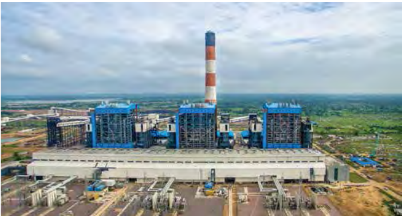
3x660 MW Lalitpur Supercritical TPP commissioned by BHEL in Uttar Pradesh
