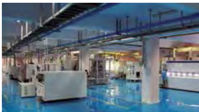
105 MW Solar PV line at BHEL, Bengaluru
