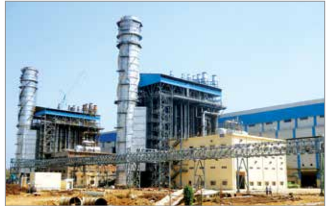
2x363 MW Gas-based Power Plant, OTPC-Palatana
