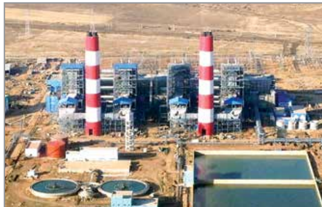
4x125 MW Kosti Thermal Power Plant, Sudan
