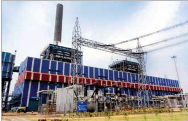
2x270 MW Adhunik TPS-Unit 1 commissioned
