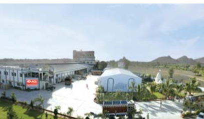
AGL Idar Plant (Floor Tiles)
