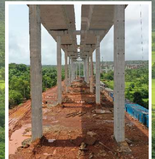
The elevated corridor consists of numerous piers that reach height of up to 40 meters.
