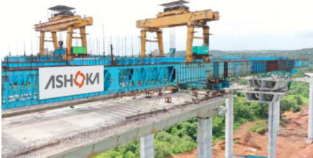
Mopa Airport Link Road
